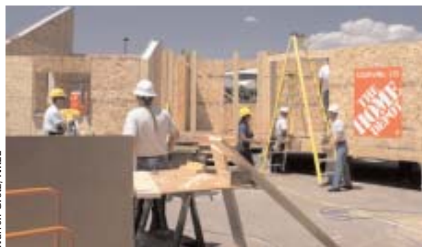
Students from the University of Colorado assembled their house at a local Home Depot and got it ready to ship to Washington, DC. Note the use of structural insulated panels to build the walls.
