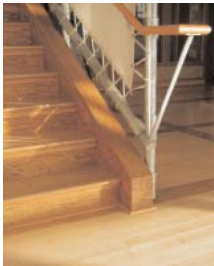
Bamboo flooring and formaldehyde-free fiberboard trim and casework are among the green building materials incorporated into the Chesapeake Bay Foundation's new headquarters.
