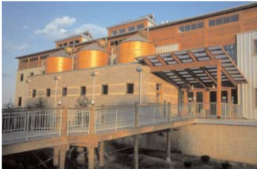
Robb Williamson Clerestory windows on the north side of the building provide daylighting for the second floor offices of the Chesapeake Bay Foundation's Philip Merrill Environmental Center. Three cisterns collect and store rainwater, which is used for most of the building's non-potable water need.
