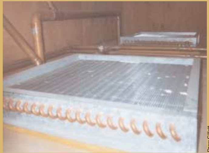
The heat exchanger was as clean as a new one after over 18 years of use.
