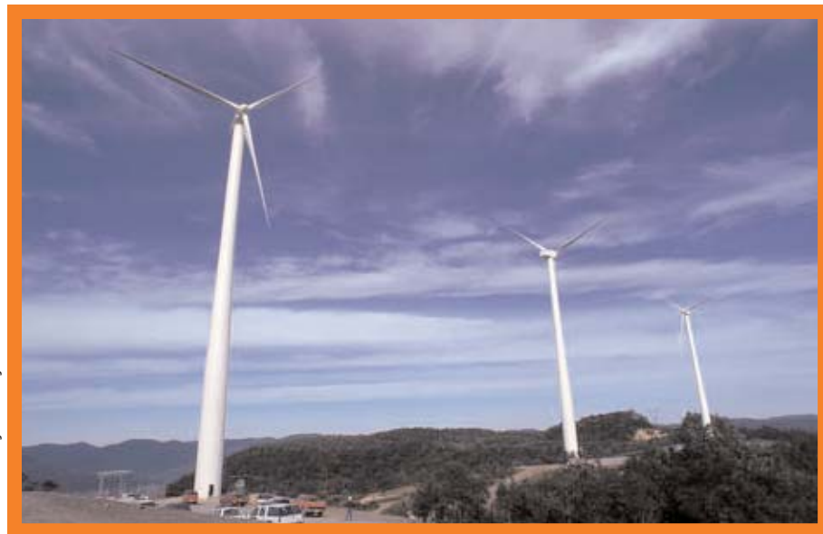
The 2-MW Buffalo Mountain Wind Project in Oliver Springs, Tennessee, features three 660-kW turbines that are part of the Tennessee Valley Authority's Green Power Switch energy program, which lets consumers buy a portion of their power from renewable energy sources. TVA plans to add 20 MW of wind power by October 2003.
