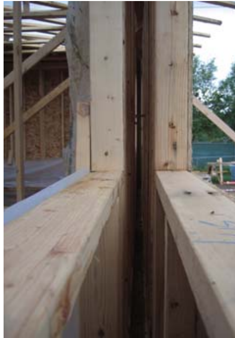
The Habitat/NREL team chose double stud wall construction (above), because it has low material costs and uses familiar volunteer-friendly techniques. Raised heel trusses (below) accommodate 2 feet of blown-in fiberglass in the attic, giving the top of the thermal envelope an insulation rating of R-60.
