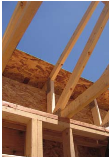
The Habitat/NREL team chose double stud wall construction (above), because it has low material costs and uses familiar volunteer-friendly techniques. Raised heel trusses (below) accommodate 2 feet of blown-in fiberglass in the attic, giving the top of the thermal envelope an insulation rating of R-60.
