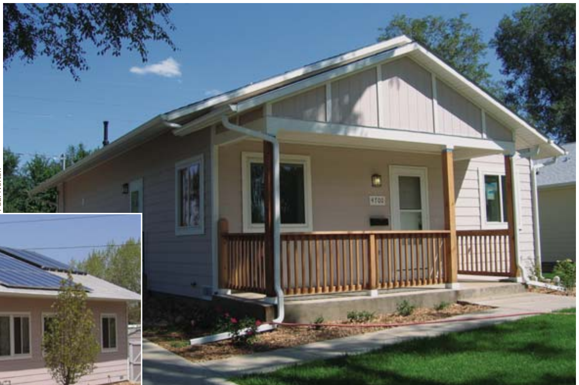
Except for the 4-kilowatt photovoltaic system and the collectors for solar water heating on the south roof, the Habitat zero energy house looks like any other Habitat home.
