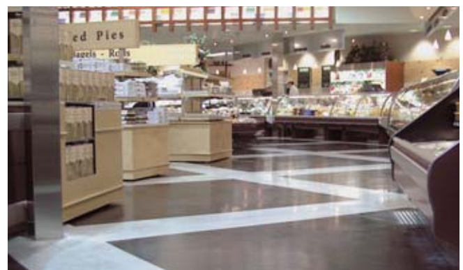
The process of polishing concrete allows a concrete slab to serve as the finished floor surface.
