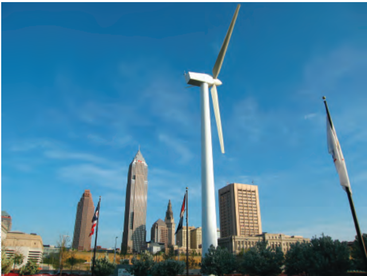
The wind turbine on the front lawn of the Great Lakes Science Center in Cleveland, Ohio, helps increase public awareness about renewable energy, and provides an estimated 7 percent of the building's annual energy needs.
