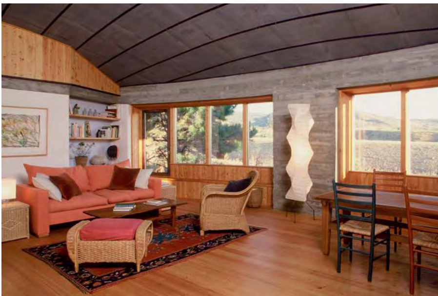
The materials in this home near Boulder are all natural, and are shown off in their natural state. Walls are adobe brick, rammed earth, or natural plaster, flooring is Colorado spruce, and the upholstery is cotton.
