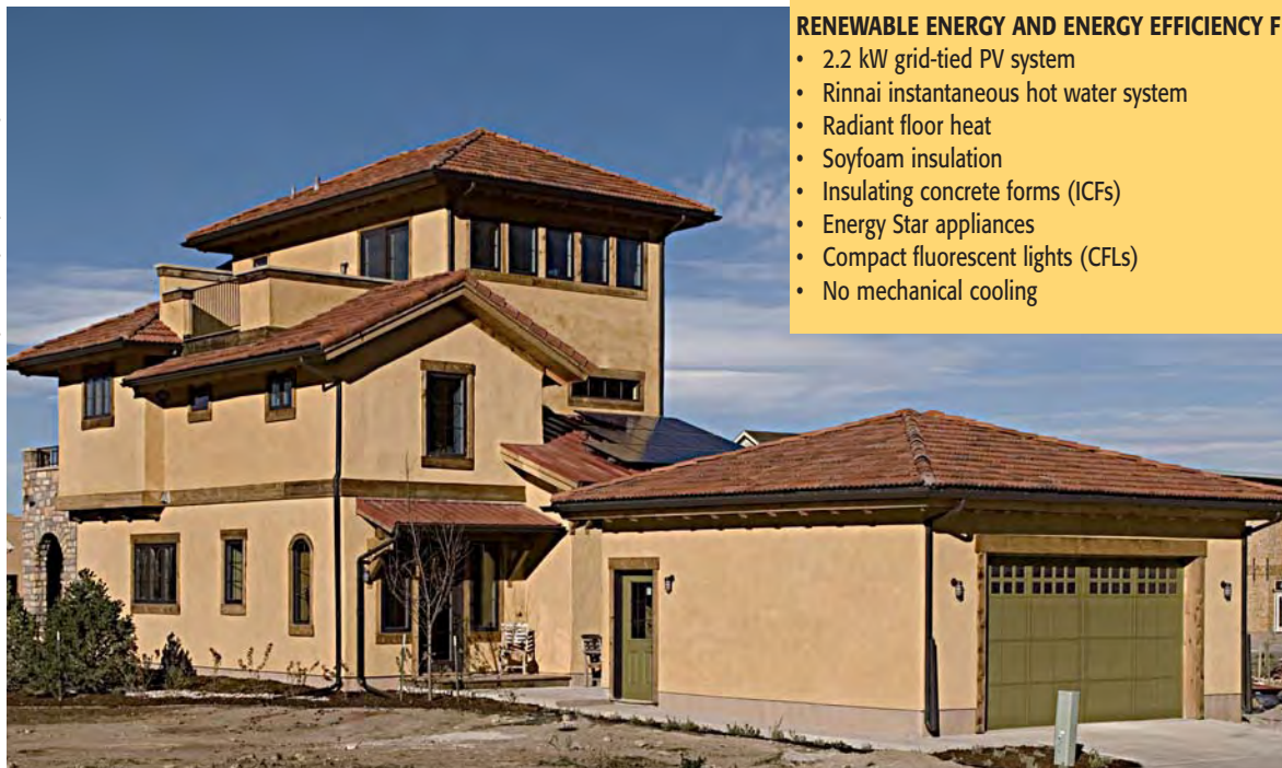
Merten Homes' new straw bale home in Old Town North in Fort Collins boasts R-28 walls, R-72 ceilings, and a 2.2-kilowatt grid-tied solar electric (photovoltaic or PV) system.
