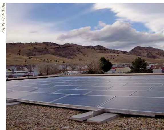
Namaste Solar Electric collaborated with the Center for ReSource Conservation to install a 10.5-kilowatt solar PV system on the Boulder Shelter for the Homeless, which supports its mission to provide safe shelter, food, and self-sufficiency services for the homeless in the community.
