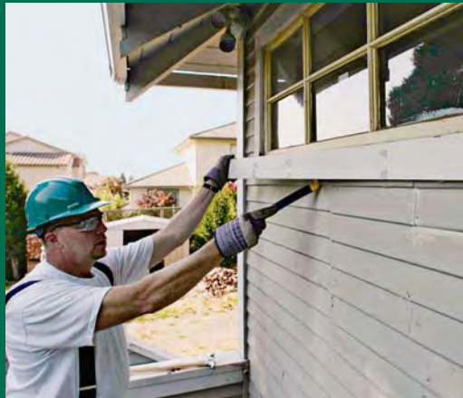
A small, thin prybar is indispensable for removing delicate trim from both the interior and exterior of a house during deconstruction.
