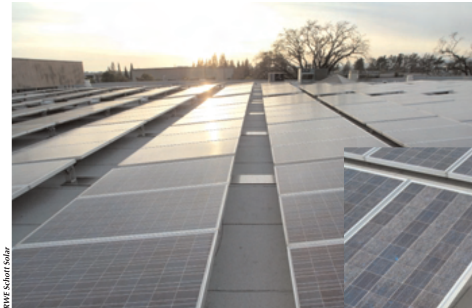
RWE Schott Solar's prototype photovoltaic system for flat roofs uses an approach that eliminates roof penetrations but stays safely secured even in very high wind conditions.
