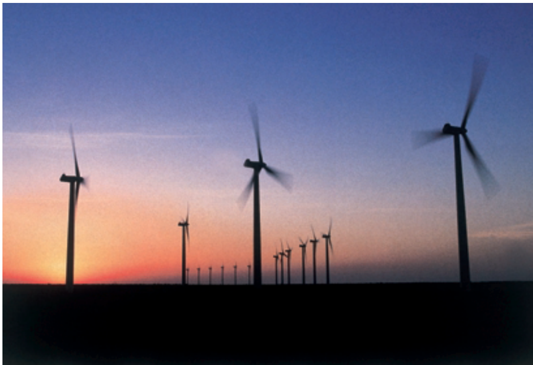
Wind turbines of the Southwest Mesa project, in McCamey, Texas, were manufactured by NEG Micon of Denmark. There are a total of 107 units producing 74.9 megawatts at this installation.
