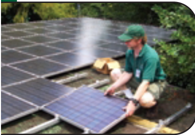
Evergreen Solar shipped 167 panels to Washington, DC for this installation.
