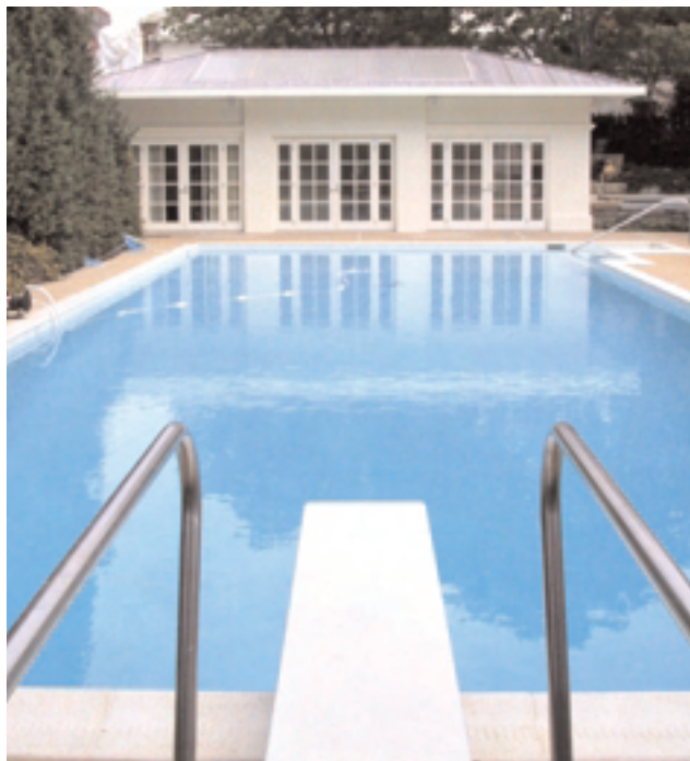
The solar thermal array on the White House pool cabana provides solar domestic hot water first to the cabana and then heats the first family's outdoor spa (at right). Any remaining solar capacity heats the pool.
