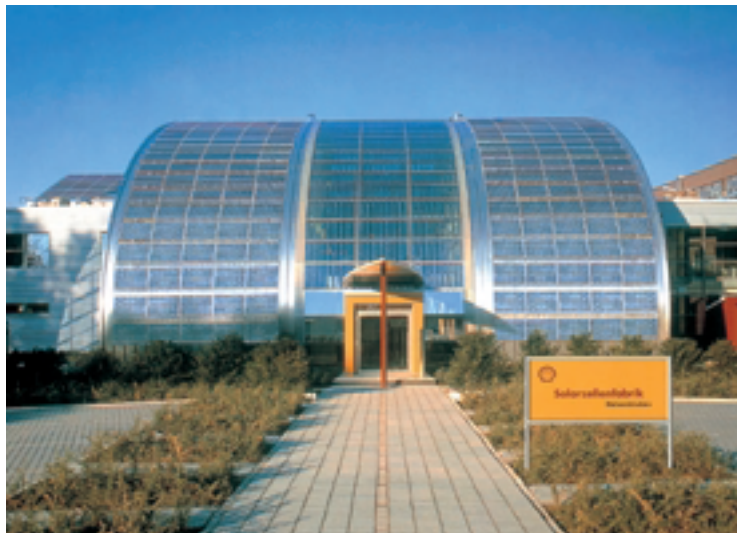
Today, Shell is one of the four largest photovoltaic manufacturers in the world. This is the Shell Solar factory at Gelsenkirchen, Germany.
