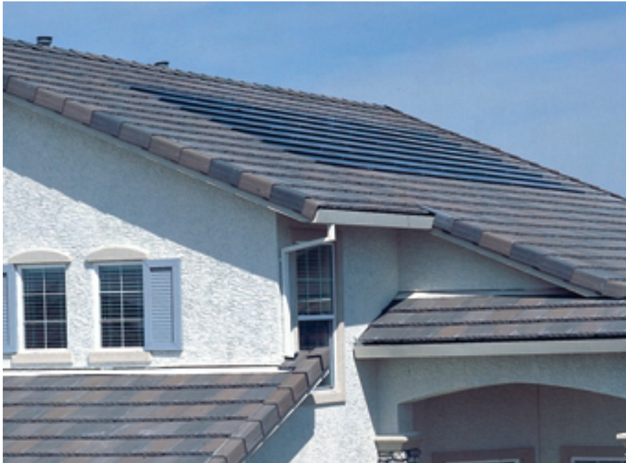
At this subdivision in Lincoln, California, roofing equipped with solar electric cells replaces some of the concrete roofing tiles.
