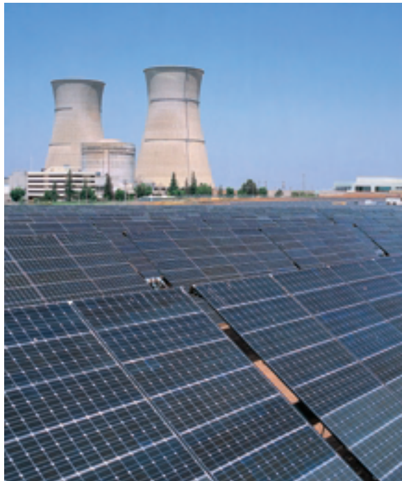
The Sacramento Municipal Utility District (SMUD) held the ceremonial groundbreaking for the photovoltaic system on the grounds of the Rancho Seco nuclear power station site in October 1982. The site now features more than 3.9 MW of photovoltaics.
