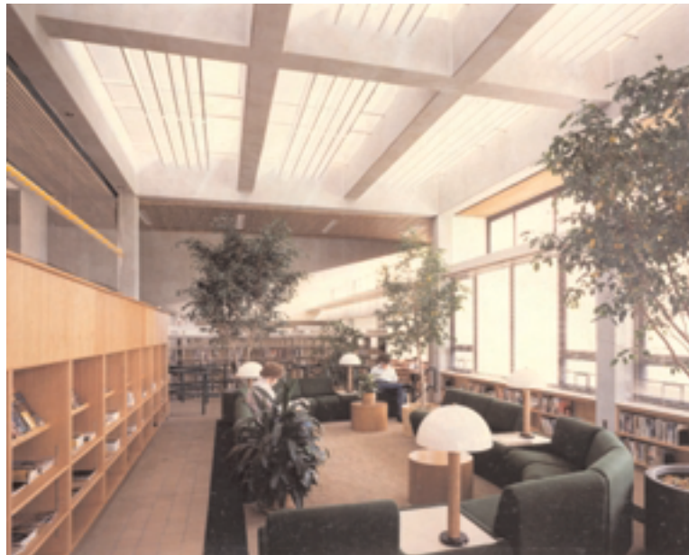
The Mount Airy library, in Mount Airy, North Carolina, a U.S. Department of Energy demonstration project built in 1981, is a completely daylit, passively heated and cooled facility that uses 75 percent less energy than a typical library in the region.
