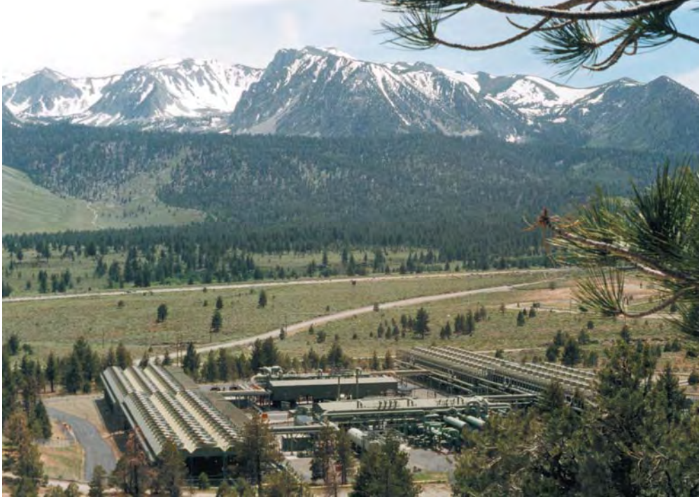
The Mammoth Lakes Power Plant is located in a picturesque area of northern California. Binary-cycle geothermal power plants release no carbon dioxide or water vapor plumes and blend into the environment.
