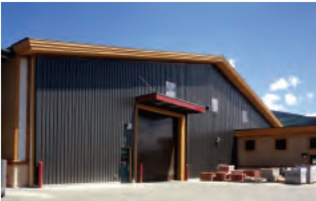
DOE/NREL, PIX 09173, Jim Yost
