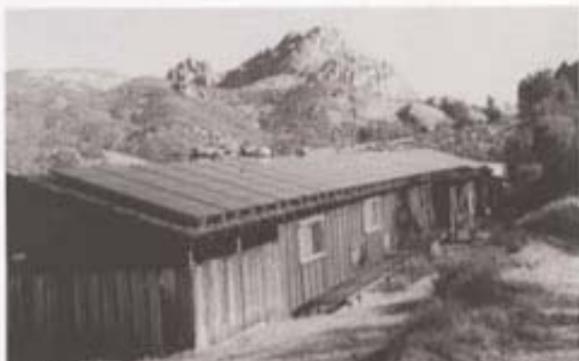
This quiet, unobtrusive hybrid photovoltaic system provides the Chapparal area on the west side of Pinnacles National Monument with clean, reliable electricity. In this pristine area, the photovoltaic installation eliminates park service staff concerns about fuel spills or leaks, because the PV system requires no fuel and produces no emissions.
