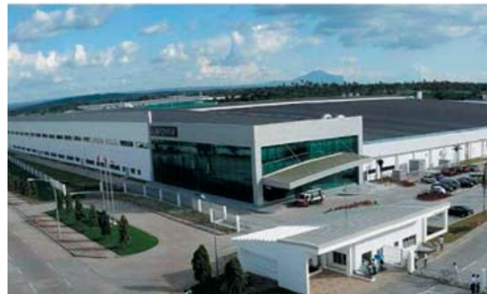
SunPower's manufacturing facilities in the Philippines produces the world's highest-efficiency solar cells while reducing the carbon footprint by 50%.
